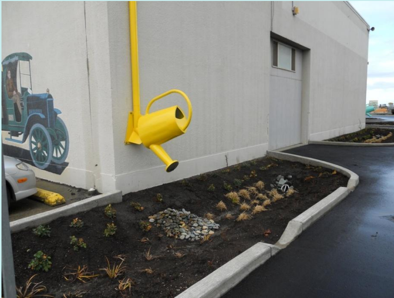
Rain garden at Port of Anacortes facility in Skagit County
